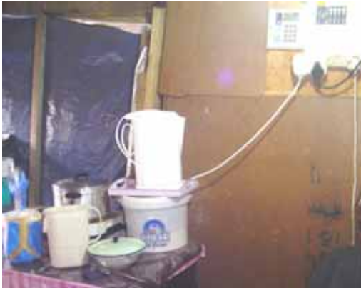
Photo 5: Kettle on unstable surface
