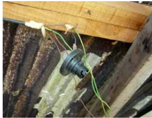
Photo 6: Unsafe wiring
